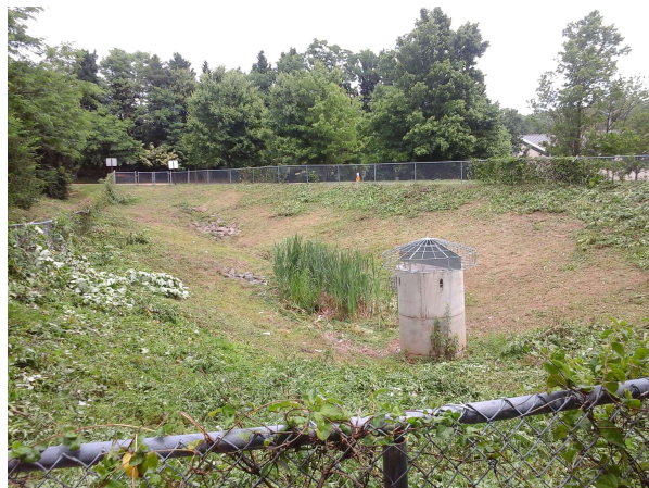
Interior of existing pond showing high flow riser
