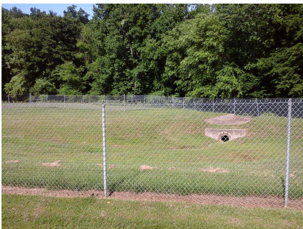
Existing dry pond and outlet configuration
