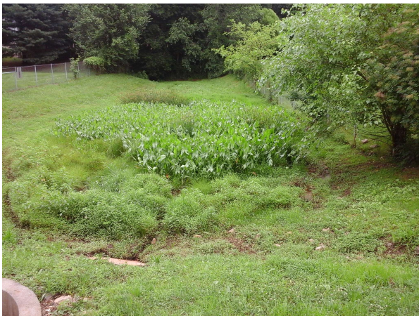
View of stormwater pond upstream of riser
