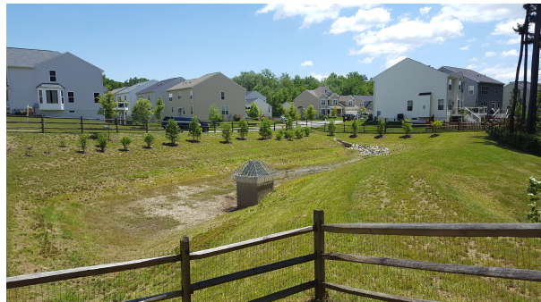
Overall view of dry pond facility
