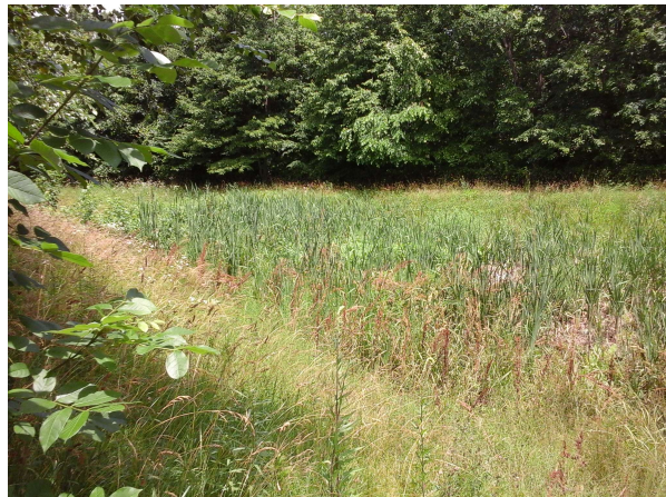
Oblique view of interior of dry pond
