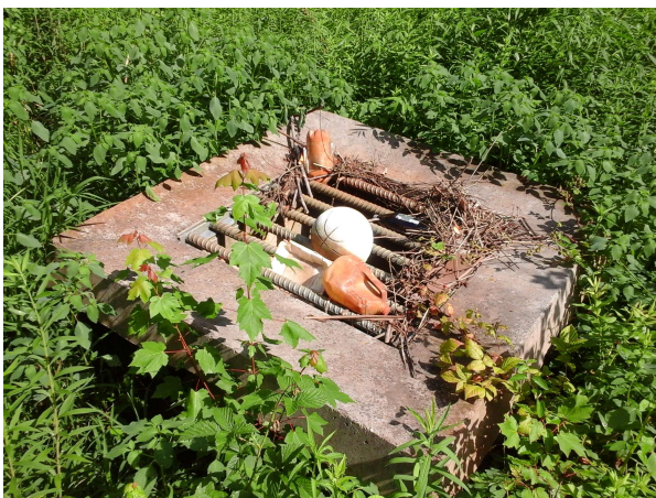
Existing high flow outlet
