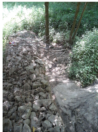
Gabion basket between stormwater outfall and riser
