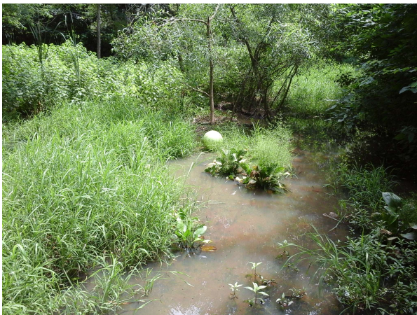
Standing water within dry pond facility
