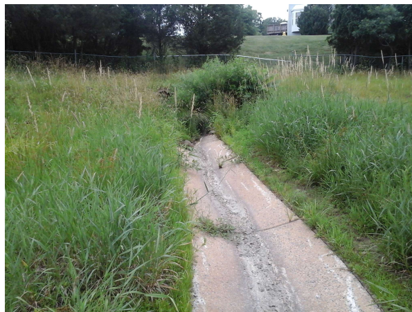
View of concrete leader channel within dry pond
