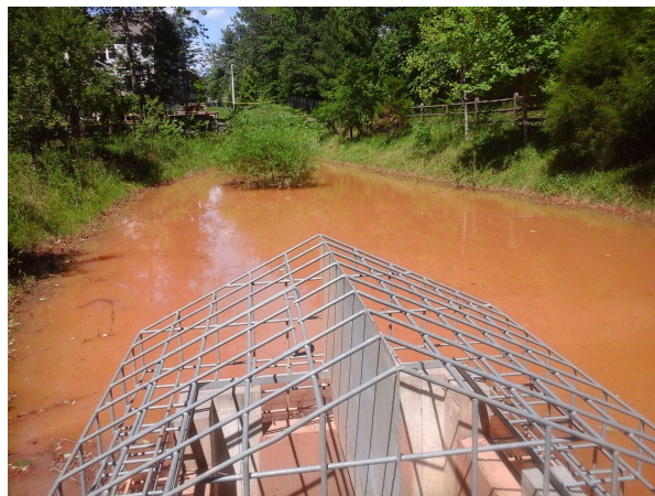
Interior of dry pond facility showing accumulation of construction site runoff
