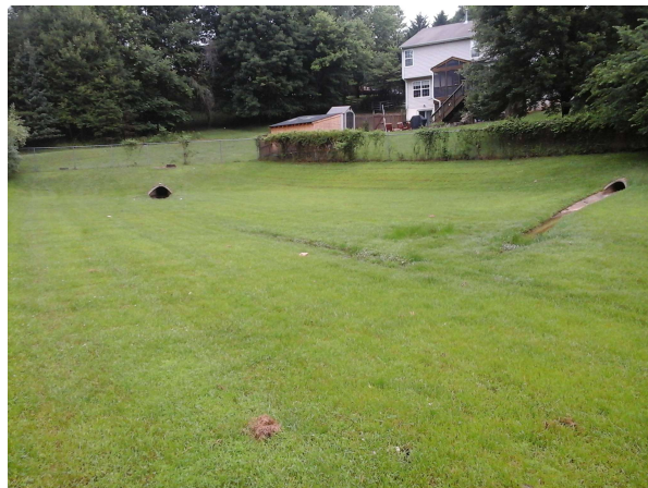
View of outfalls from stormwater network into pond.
