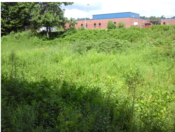
View of dry pond with middle school in background
