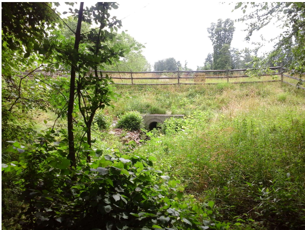
Outlet orifice of dry pond
