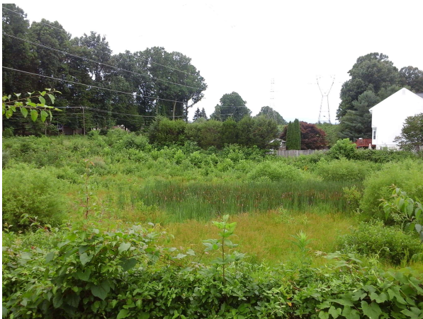
Interior of dry pond showing extensive vegetation
