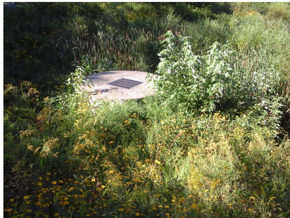
Existing outlet riser of dry pond
