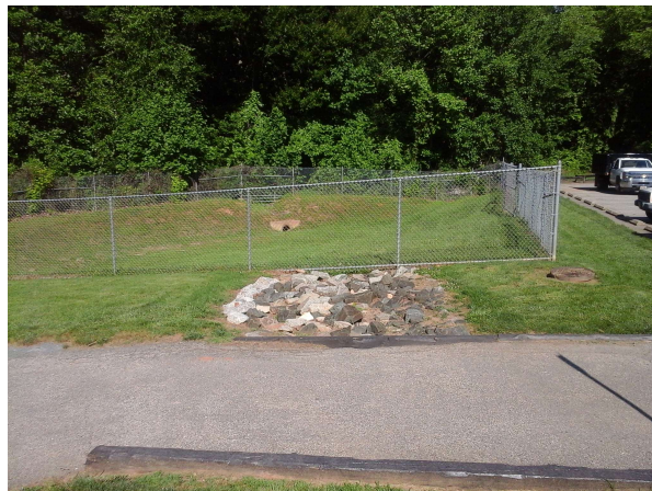
Riprap-lined channel on east approach to stormwater pond
