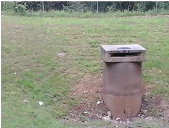
Existing riser of dry pond
