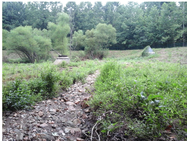
Dry pond interior, showing sanitary sewer manhole and riser
