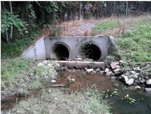
Outlet of existing facility showing low flow weir
