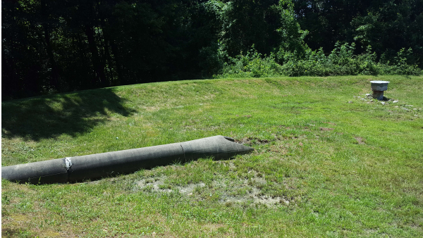
Storm drain outfall and riser of dry pond
