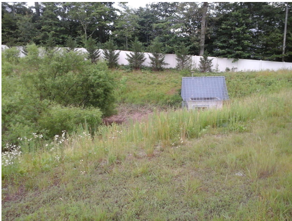
Riser of dry pond facility
