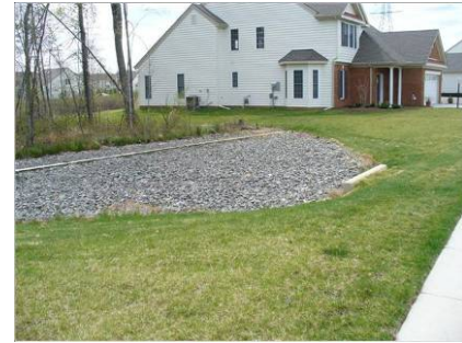
FIG 19: Henrico County has Shown Level Spreaders to be Very Effective at Eliminating Scour at Outfall Locations
