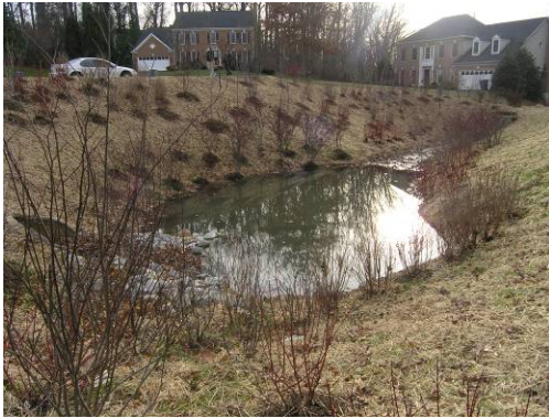
FIG 15: Northern Virginia Pond Retrofit Shortly after Construction
