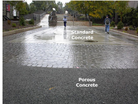
FIG 16: Side by Side Comparison of Standard Concrete and Porous Concrete at Villanova University
