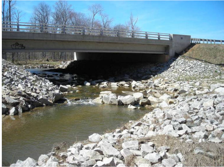
FIG 6: Existing Spriggs Rd. Bridge – Built Since Hydraulic Study
