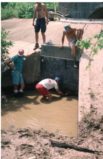
FIG 20: Construction of the Dale Blvd Retrofit project
