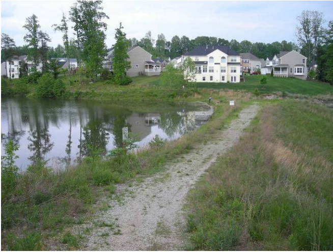
FIG 3: The embankment and outlet structure for Lake Terrapin
