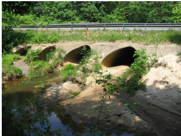
FIG 11: Downstream face of culverts under Minnieville Road (Rt. 640)
