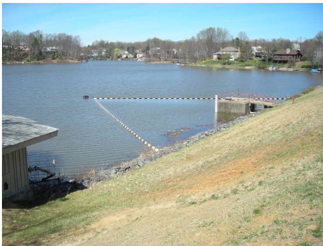
FIG 2: Outfall structure at the Lake Montclair Dam
