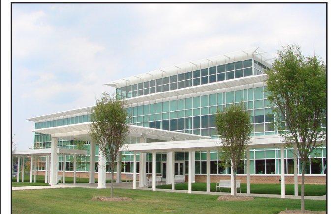
Development Services Building
