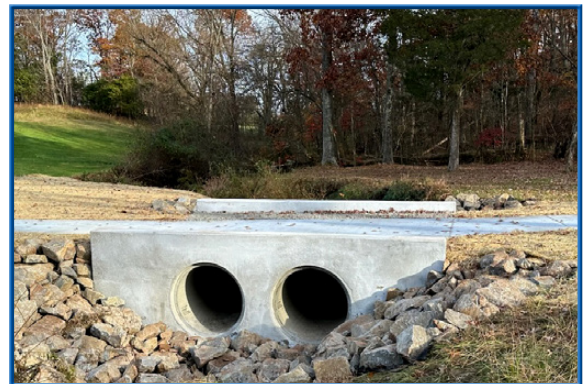
Prince William Golf Course Culvert Repair
