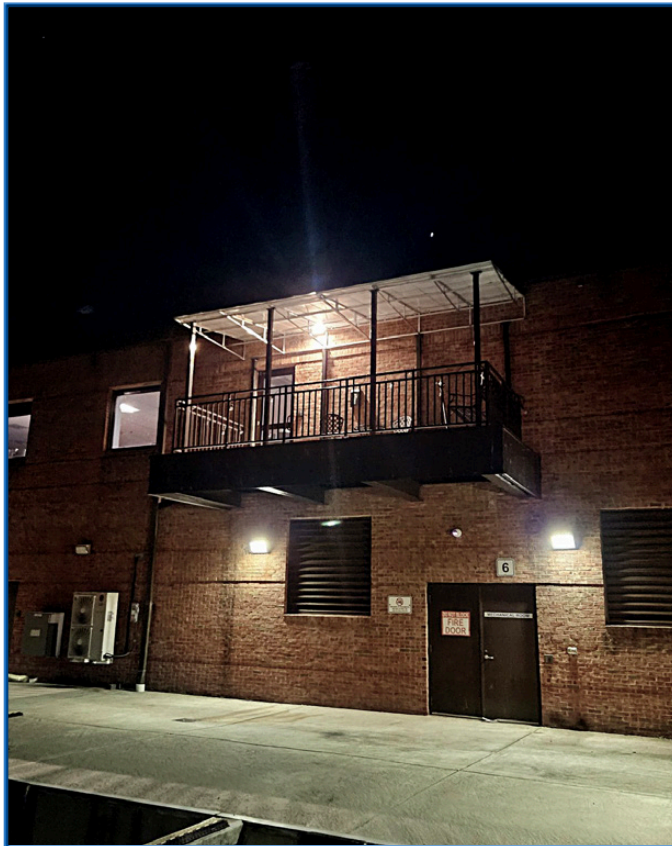
Owens Building Balcony Repair
