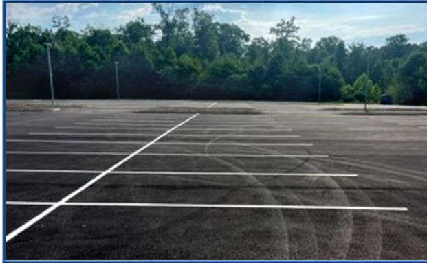
Catharpin Park Parking Lot Paving
