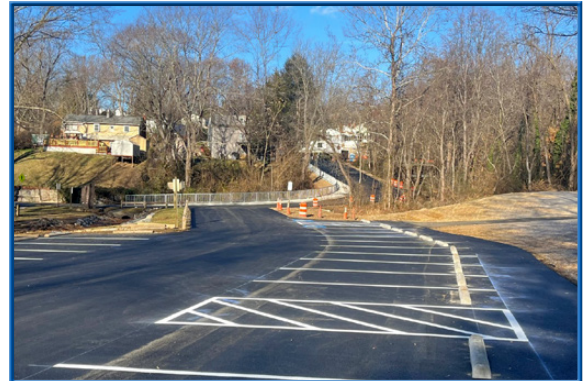
Cloverdale Park Site Improvements
