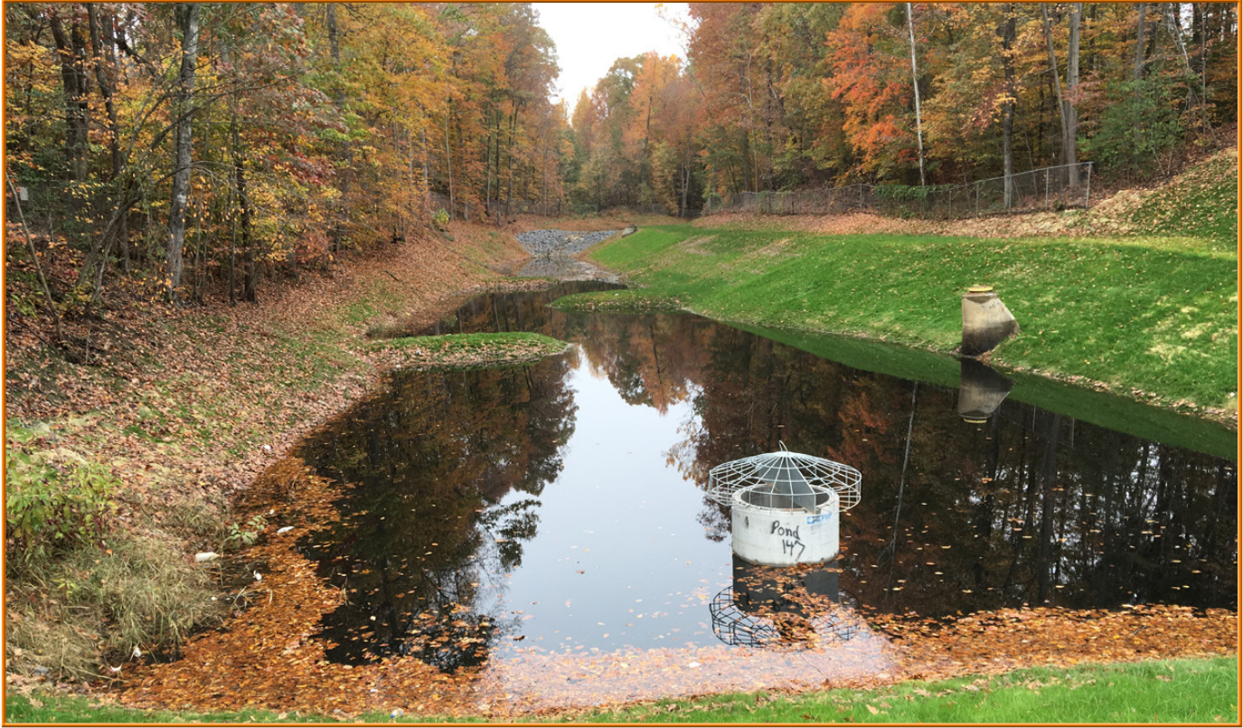
Powells Creek Watershed Water Quality Retrofit
